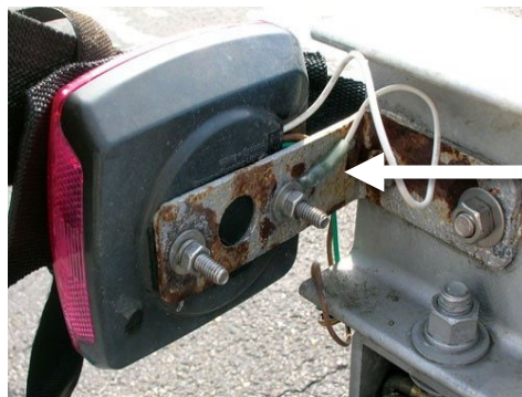
Ground wire on trailer taillight connecting the circuit to the ground, which is the trailer's frame.
